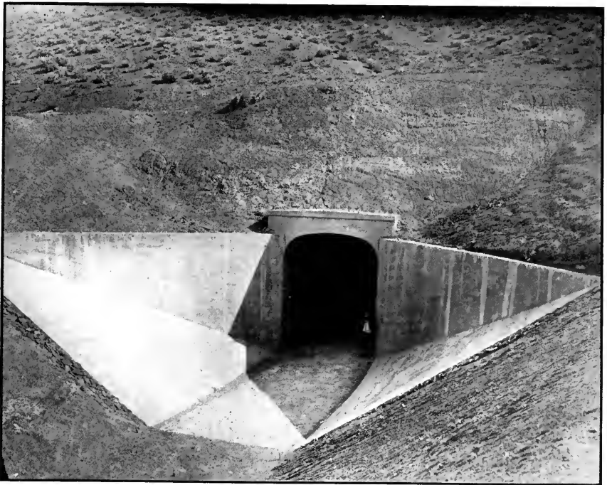
ENTRANCE TO TUNNEL NO. 1, TRUCKEE-CARSON PROJECT
